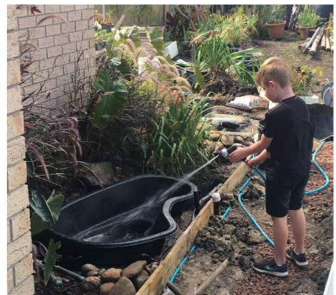
Filling the pond with water. The best way is to put a small amount in the bottom and level it out. Then fill slowly and keep adjusting the level to make sure it's right.
